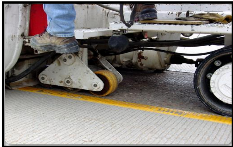
Figure 2-6: Slurry Recovery Vacuum on Texture Planer
