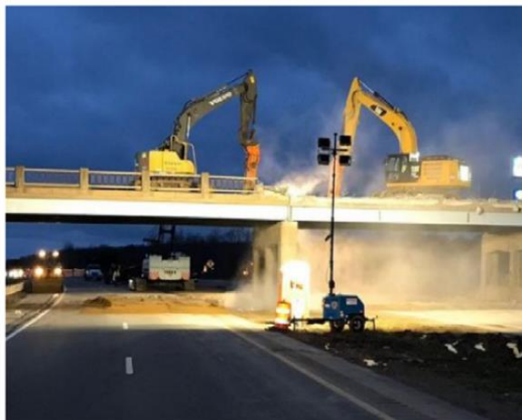
Figure 1-4 Bridge Demolition Activity Over a Large Roadway
