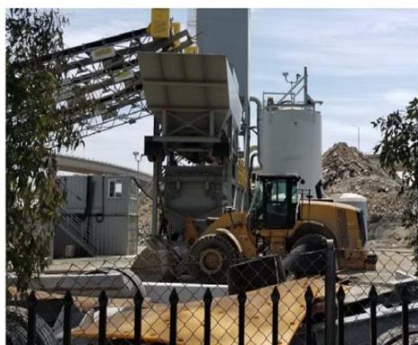
Figure 1-3 Portable Crusher at Roadway Project Near a Receptor
