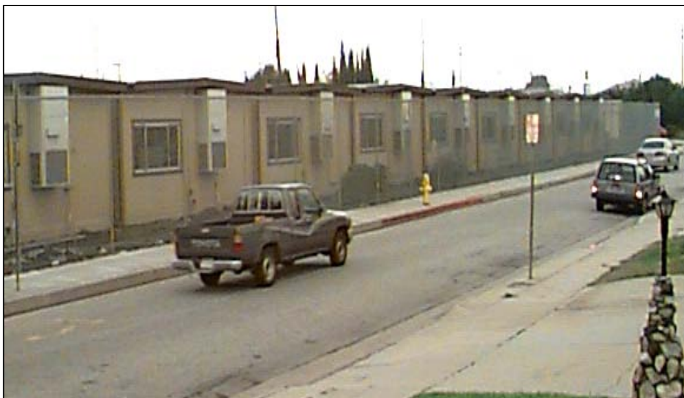
Vehicle traffic near air intakes of classrooms can be a major source of small particles, volatile organic compounds, and other pollutants.
