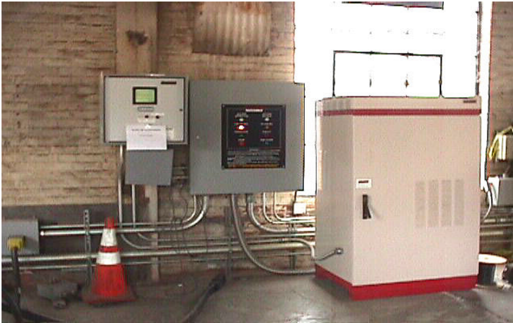
Fig. 1. eTec SuperCharge fast-charging system (33 kW) used in pack cycling.
