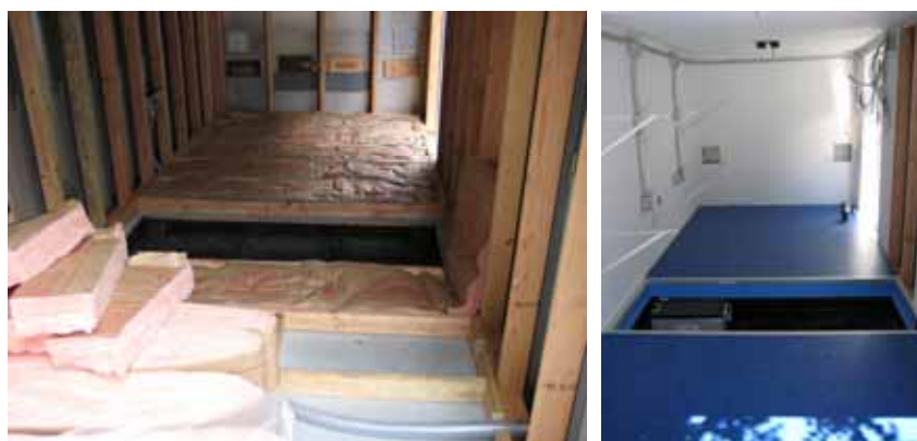
Figure 3. During construction of the Mobile Emissions Laboratory, insulation (RU-13) was added inside all walls to allow for long- term operation in extreme environments. Deep cycle marine batteries mounted under the floor provide DC power for applications where AC power is limited.
