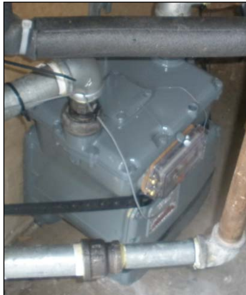
Figure 1-7: American AC-360 Gas Meter
