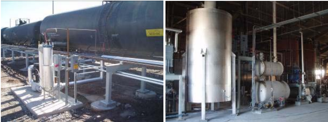
Figure 13. Accu Chem’s Trans-Loading Facility (left) and Biodiesel Refinery (right)
