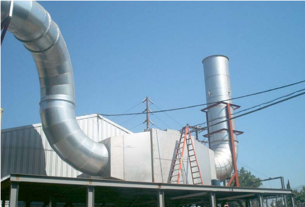
Figure 11 Photograph of Scrubber Installed by Project Team
