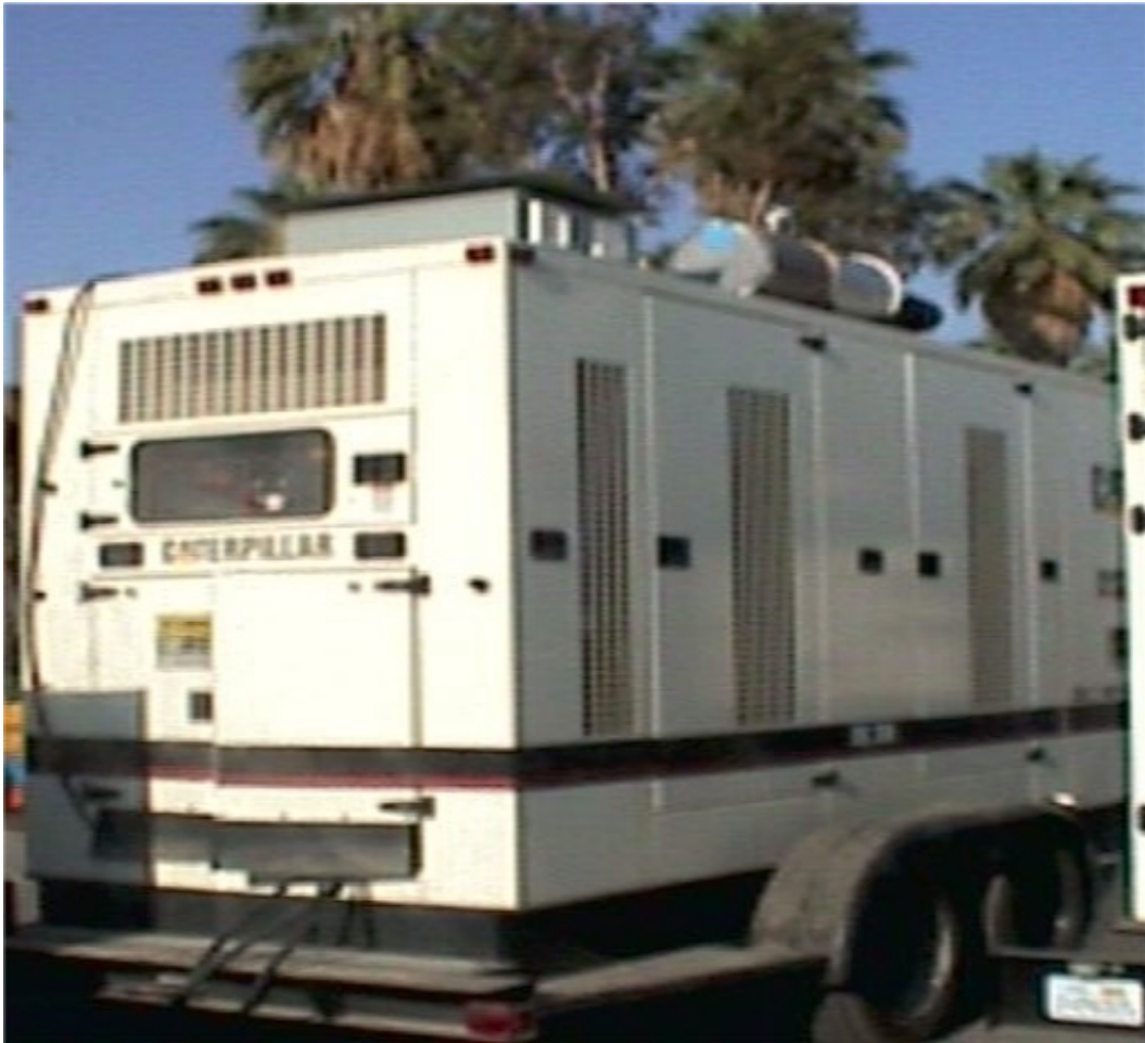
Picture 3: The 350kW installation.
