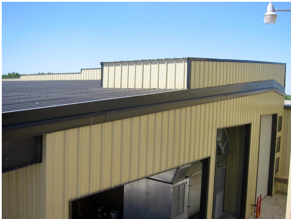
Figure 11: Roof mounted panels, raised roof collection plenum & duct to dryer fan inlet
