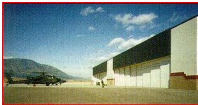
Figure 2: Example of SOLARWALL® panel heating a military building
