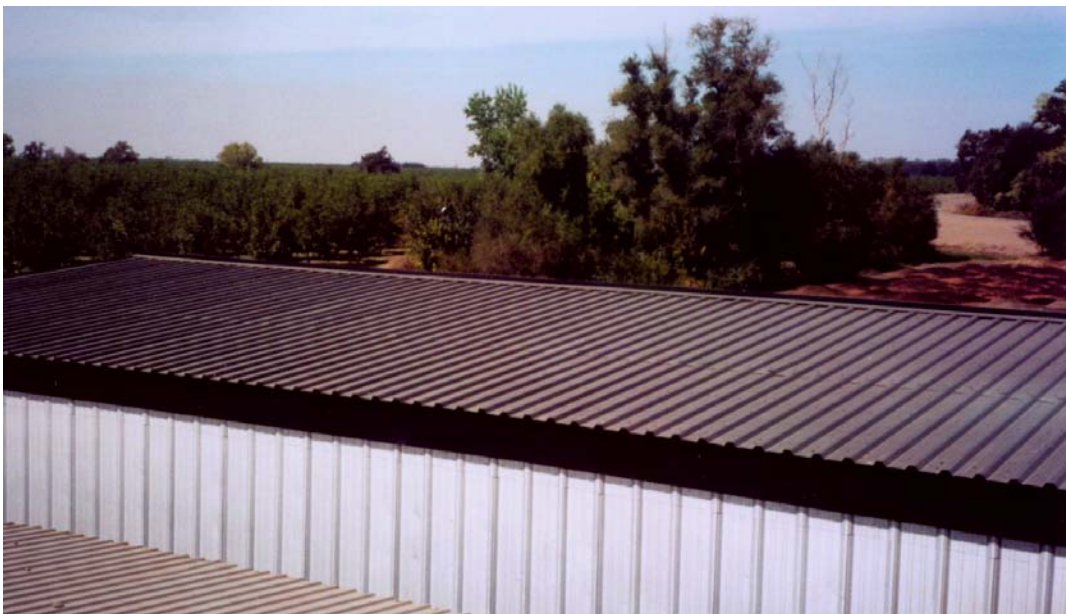
Figure 9: SOLARWALL panels on roof of dryer building
