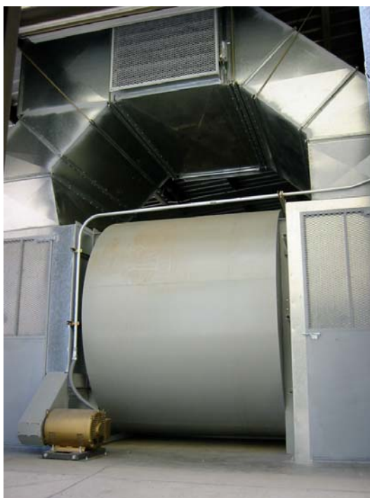
Figure 12: Solar ducts connected to two sides of 65,000 cfm dryer fan
