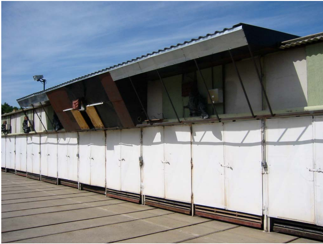
Figure 5: Dryers with roof mounted SOLARWALL panels connected to air intake
