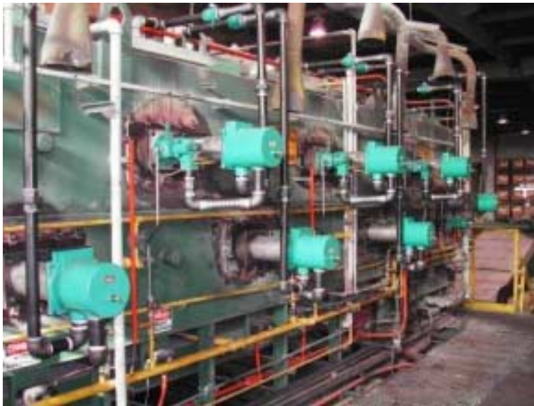
Figure 12. Installed FIRB's on ITW's Heat Treat Furnace #15
