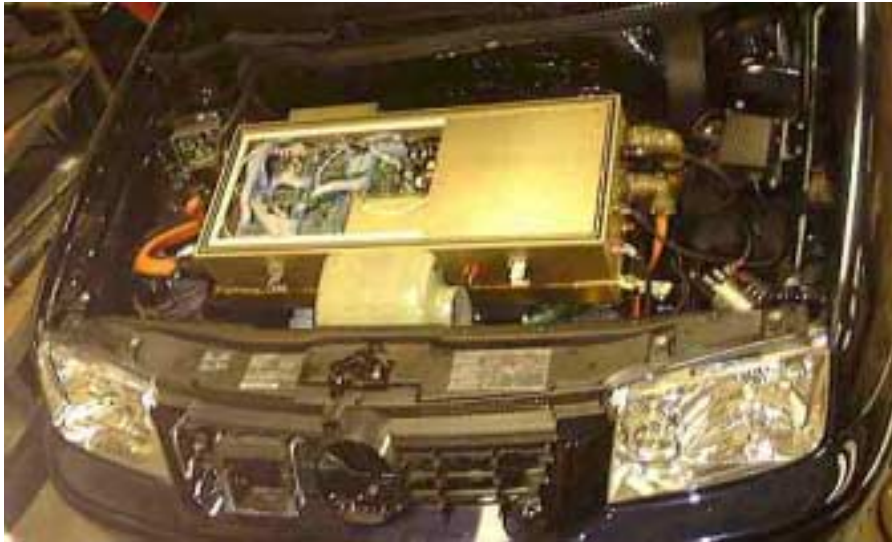
Figure 3. Electric Drive System Installed
