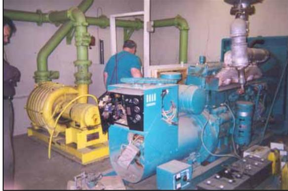
**Figure 33. 25 Hp blowers (yellow in background) and existing diesel gen set (foreground).**
