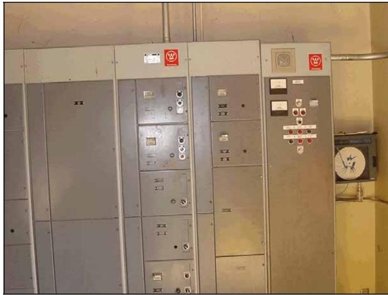
**Figure 47. Treatment Plant Switching System**
