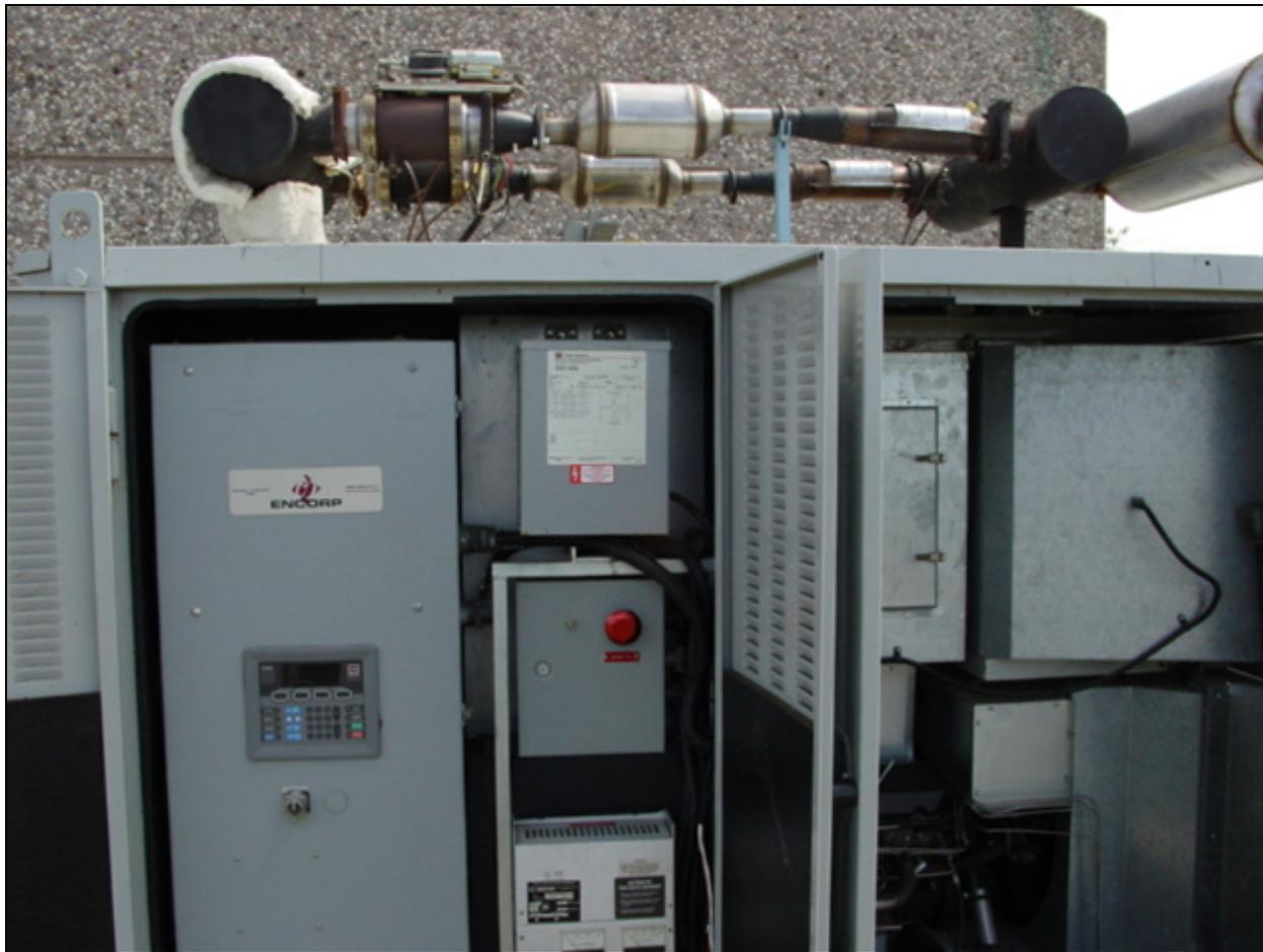
**Figure 59. MicroNOx Exhaust System Installed For Field Testing.**
