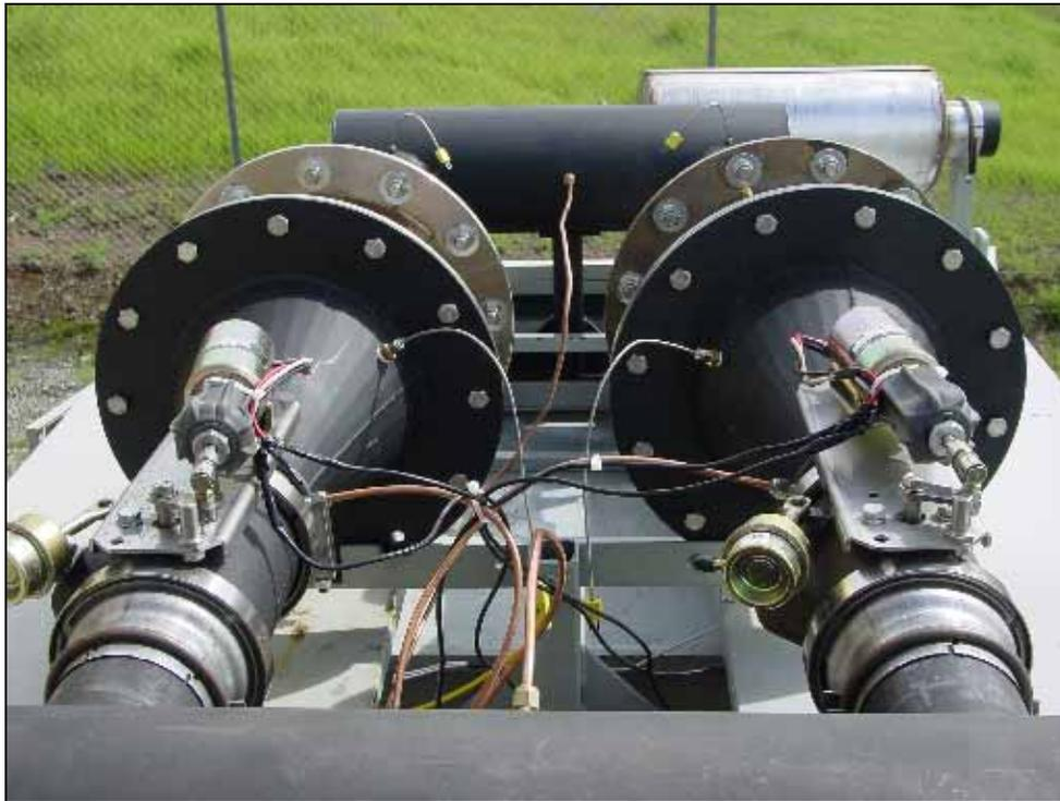
**Figure 39. NOx Reduction Catalytic Sections And Exhaust Flow Control Valves.**
