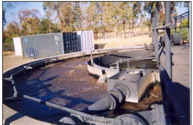
**Figure 32. Aerobic Digester.**
