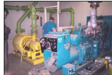
**Figure 4. 25 Hp blowers and existing diesel gen set**
