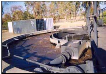
**Figure 3. Aerobic Digester.**
