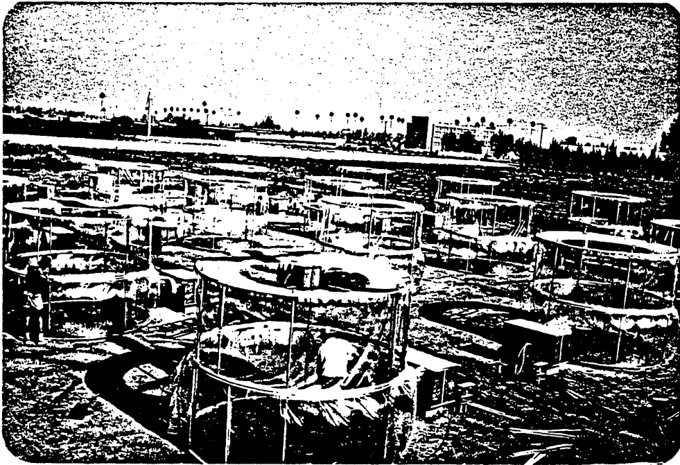
Figure 1. ARB Fumigation Facility at University of California, Riverside, being completed. Note blower housings and activated charcoal filters at right of greenhouse in immediate foreground. All sampling and power lines are installed underground.
