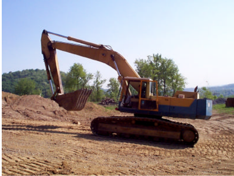
Figure 44 Excavator Hauling Operation
