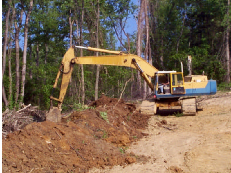
Figure 45 Excavator Trenching Operation
