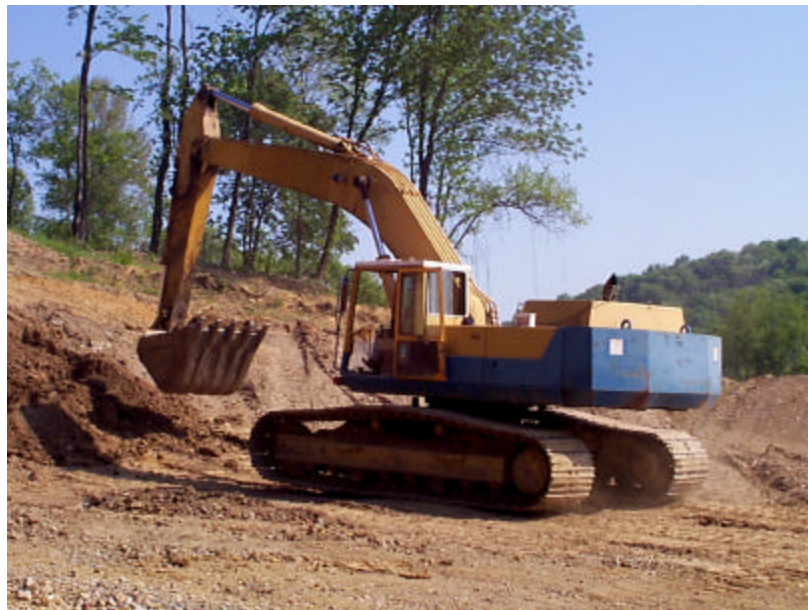
Figure 43 Excavator Digging Operation
