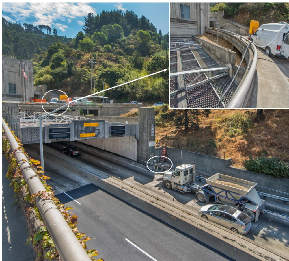
Figure 1. Instrumented van positioned on an overpass at the Caltrans facility at the Caldecott Tunnel, sampling the exhaust from a truck as it travels eastbound on Highway 24 and enters Bore 1 of the tunnel. The van is circled in the wide-view image and shown in more detail in the inset picture. The roadside camera positioned at the entrance to the tunnel is also circled.
