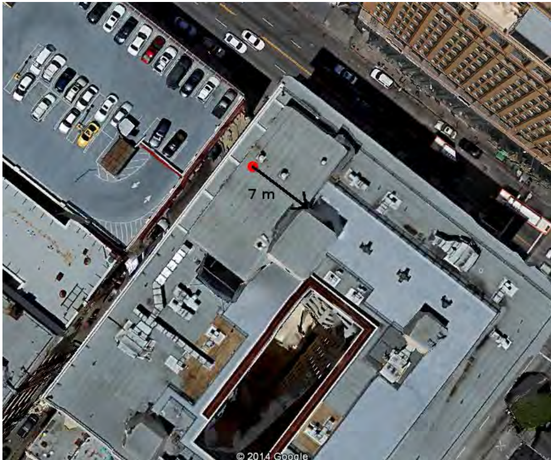
Figure A6: Location of rooftop sonic anemometer near the edge of a section of roof about 10 m above the rest of the roof. A small structure sites about 7 m to the east of the sonic.
