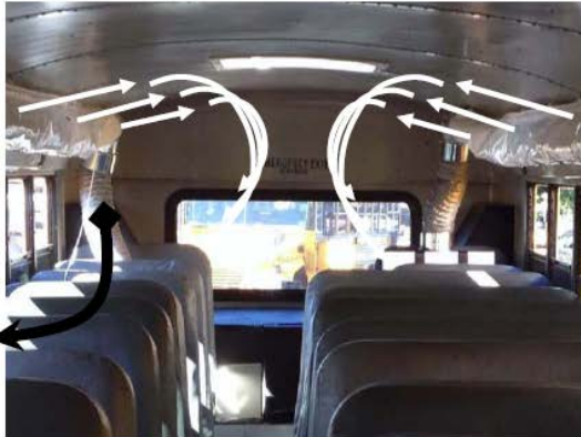
b. Air Distribution Ducts
