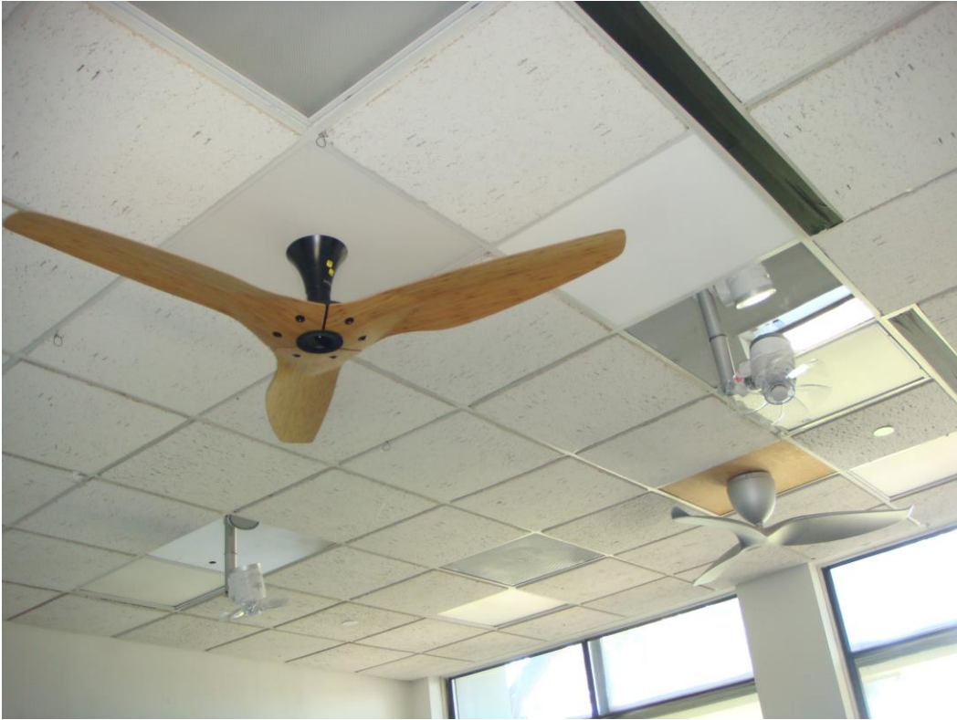
Figure 67 Four ceiling fans installed in the ceiling for testing
