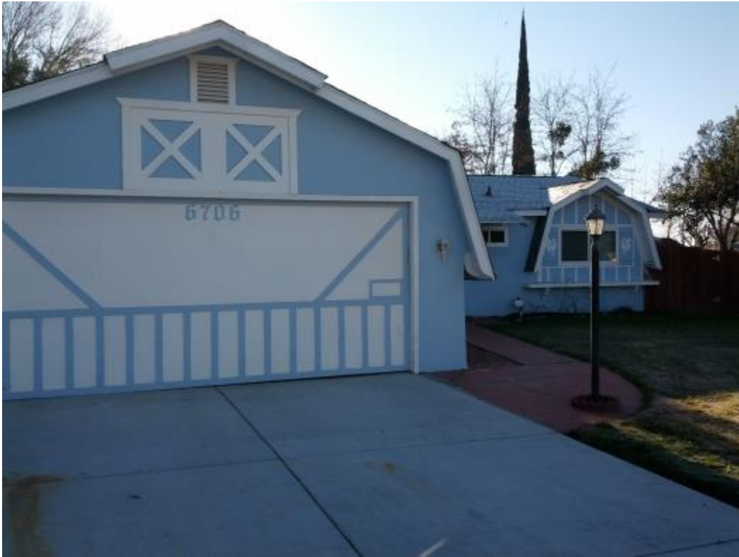
Figure 9.32. Image of front of Test House 6.
