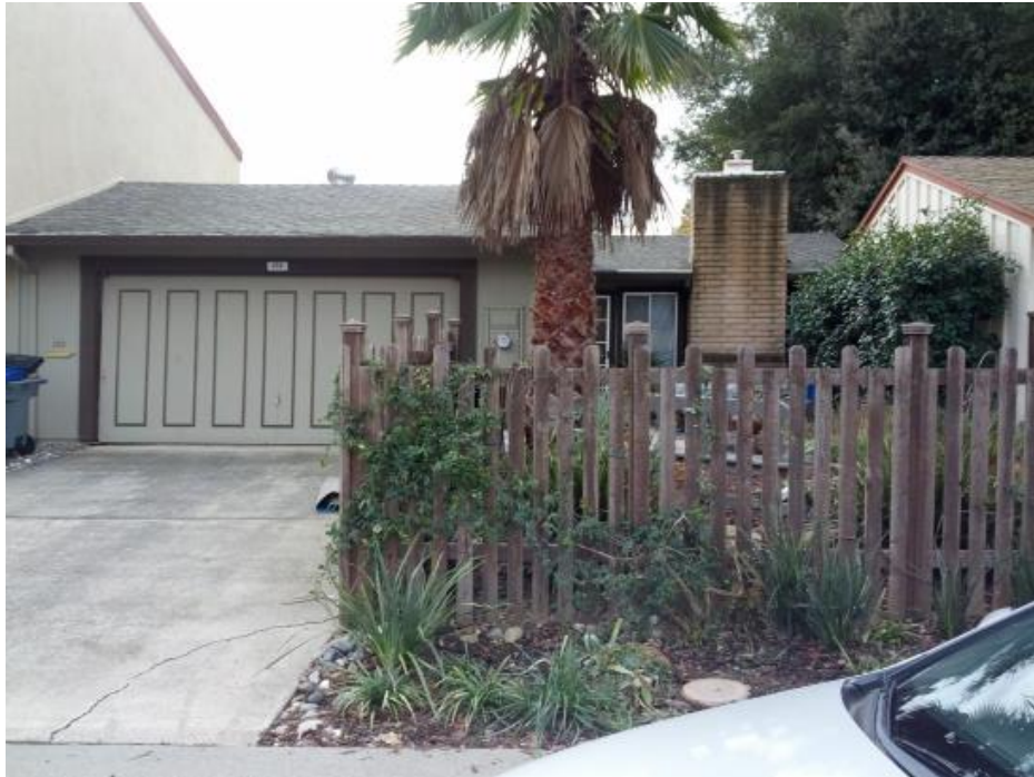
Figure 9.28. Image of front of Test House 5.
