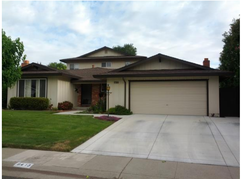
Figure 9.16. Image of front of Test House 2.
