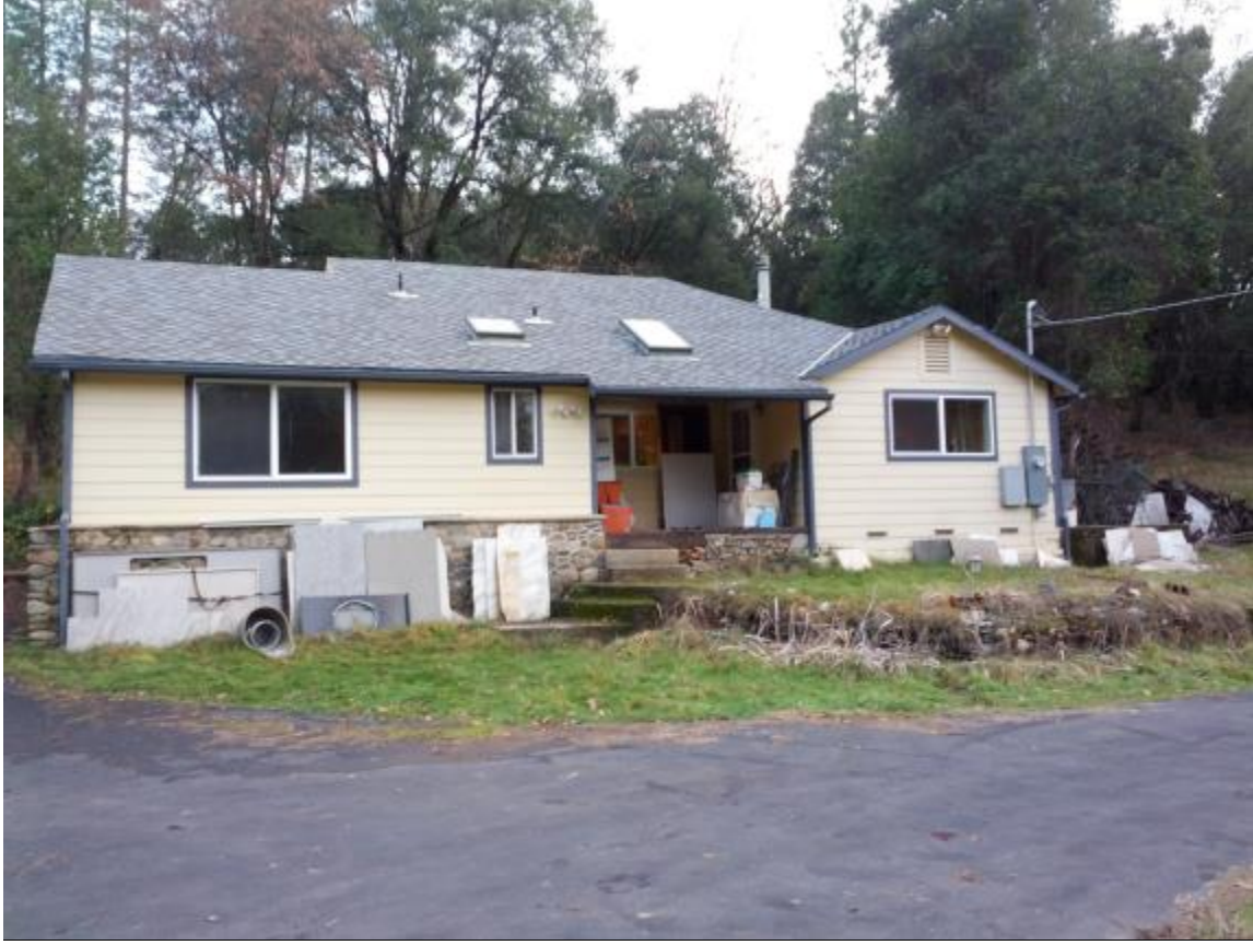
Figure 9.24. Image of front of Test House 4.
