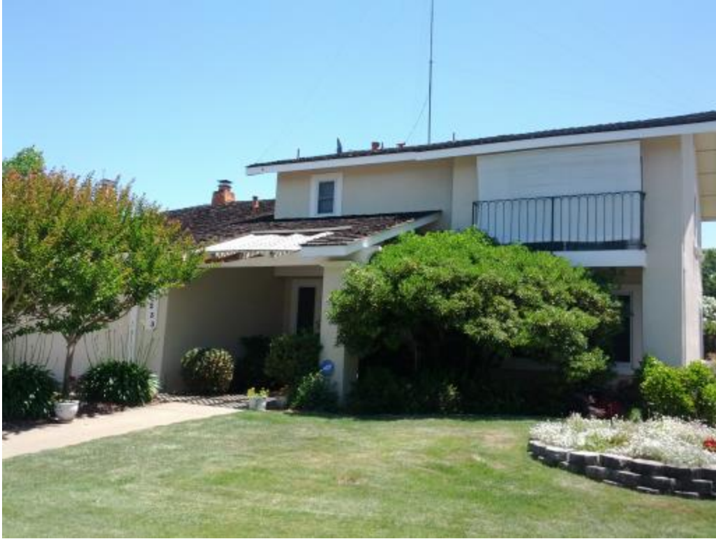
Figure 9.20. Image of front of Test House 3.
