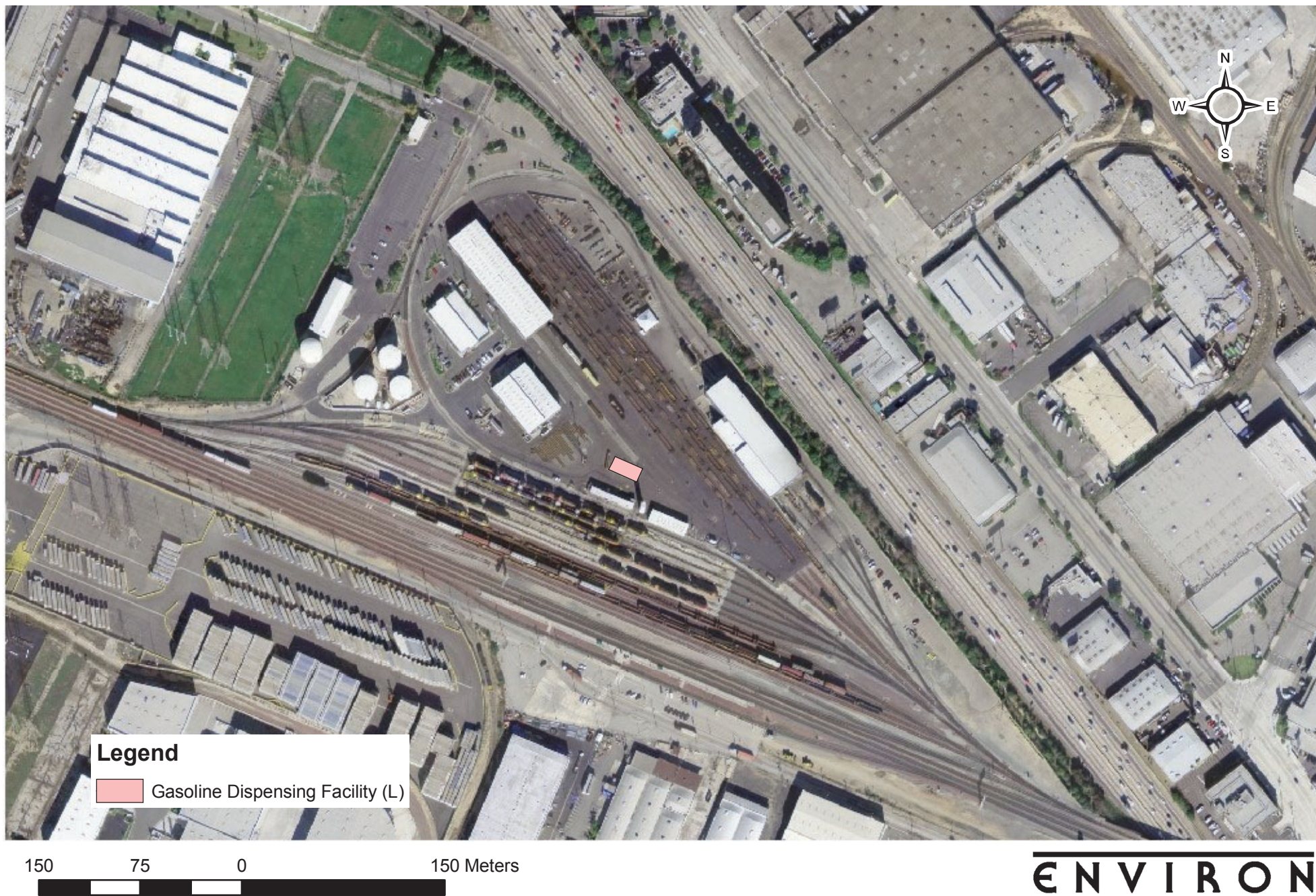
Figure 4-5: Location of Modeled Permitted Stationary Source BNSF Commerce Mechanical Rail Yard Commerce, California
