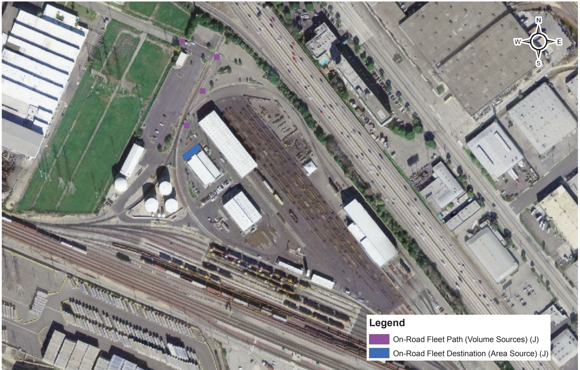
Figure 4-4c: Locations of Modeled On-Road Fleet Sources (Travel Route 3) BNSF Commerce Mechanical Rail Yard Commerce, California
