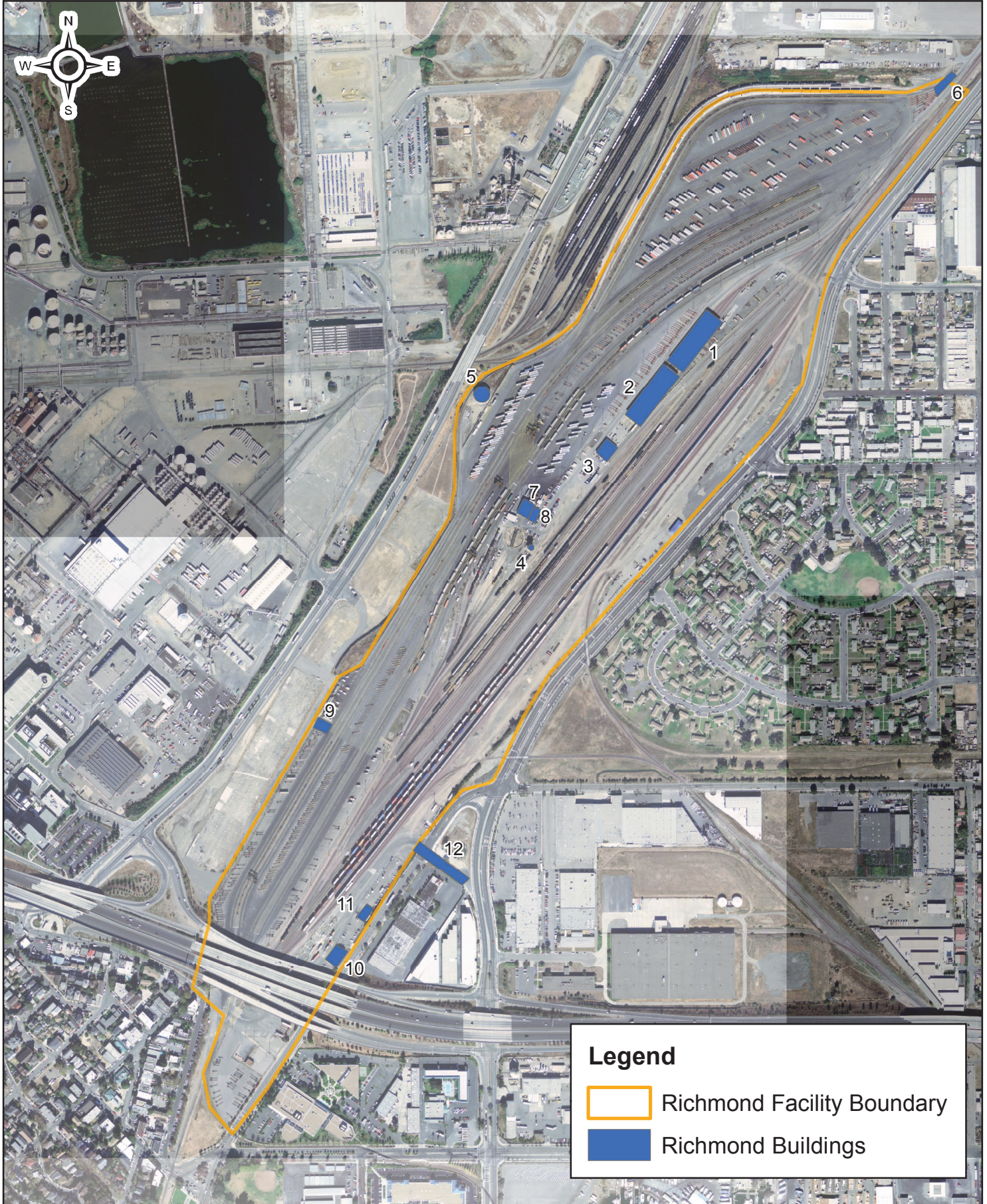
Figure 4-7: Location of Buildings and Structures at the Facility BNSF Richmond Rail Yard Richmond, California
