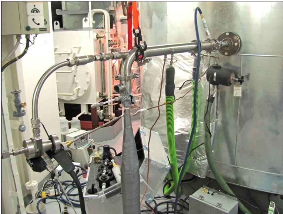
**Figure 4-3 Installed Sampling System on the Stack of the Vessel**
