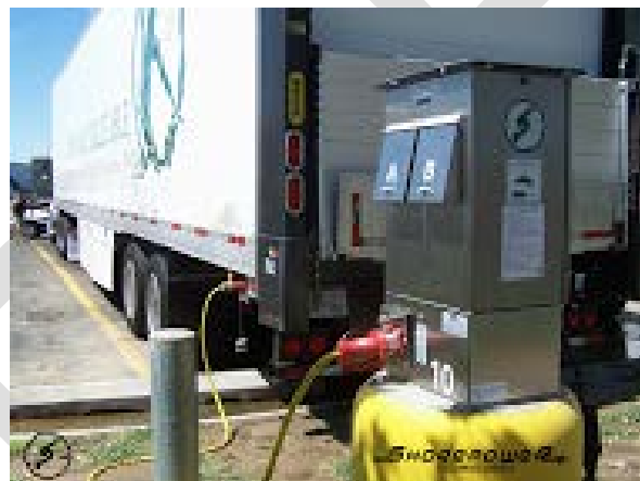
Figure III.A-4: Parking Area Power Plug Pedestal
