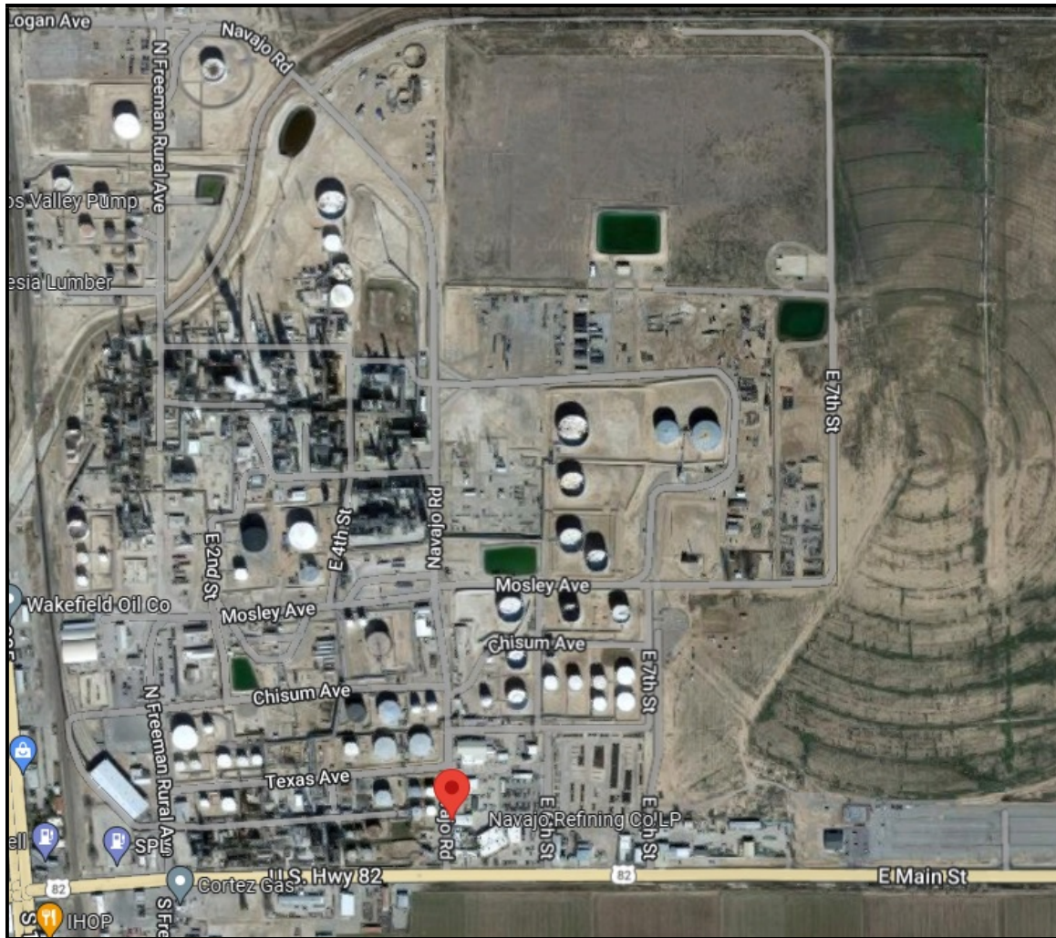
Figure 1-1 Aerial View – Artesia Renewable Diesel Company LLC
