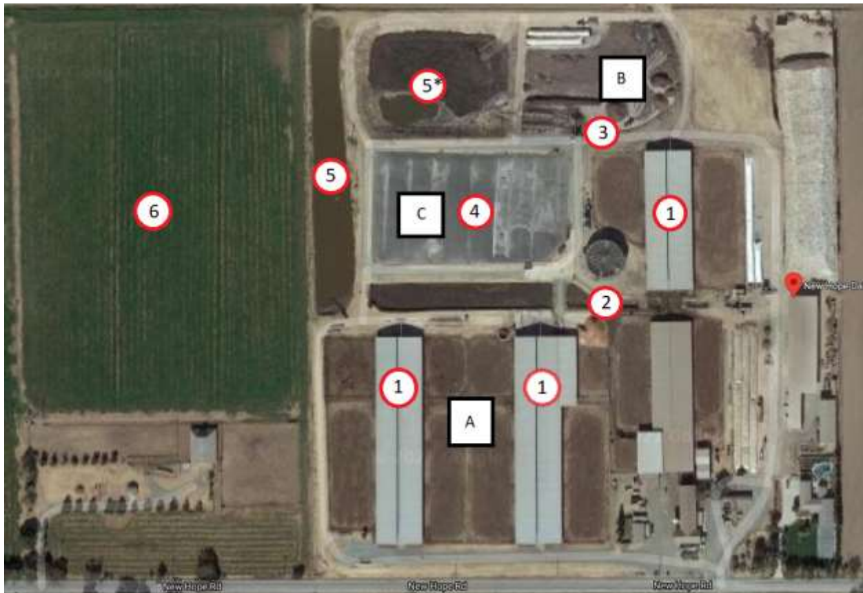
Figure 2. Aerial Image of the Dairy Farm and Covered Lagoon Digester
