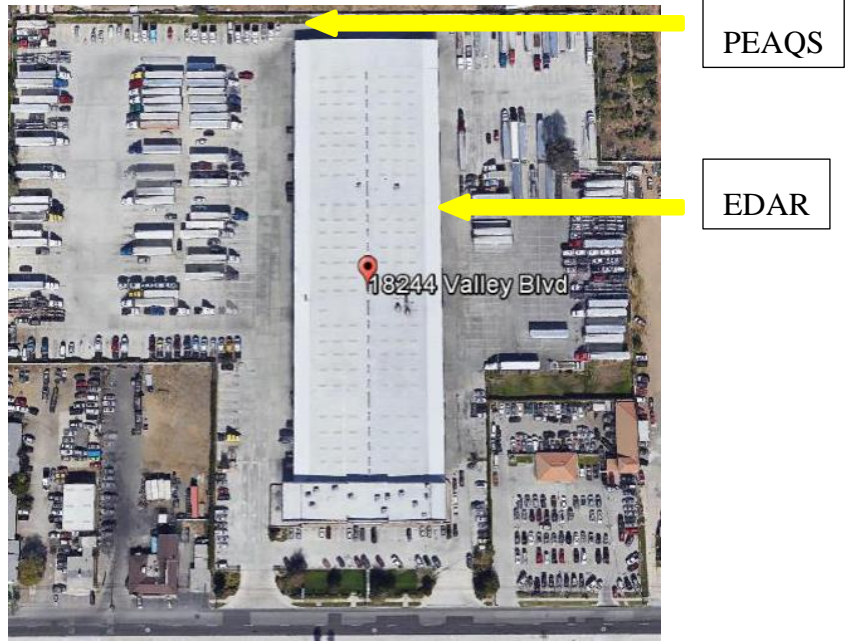
Figure 3-4 Overview of J&R Facility and positioning of EDAR and PEAQS systems
