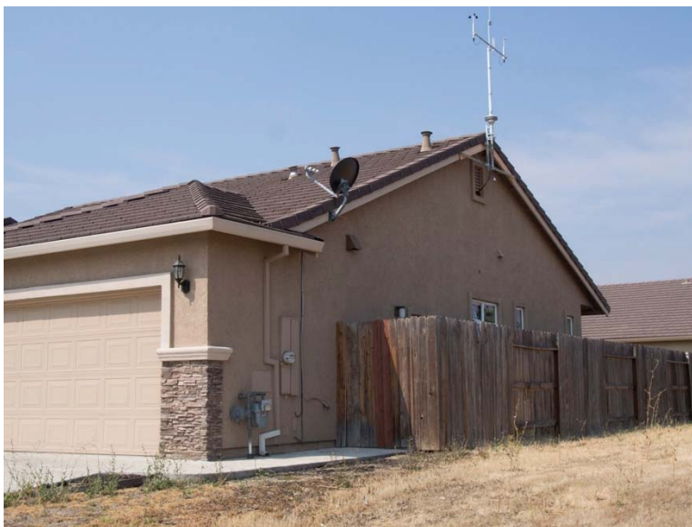
Figure 2.12. Weather station and air intakes for supply ventilation and outdoor particle sampling.
