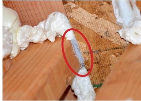
Sealed leak in between manual caulk application at the Honda Smart Home
