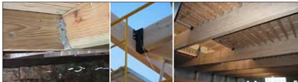
Figure 8-28. Typical joist hanger connectors.
