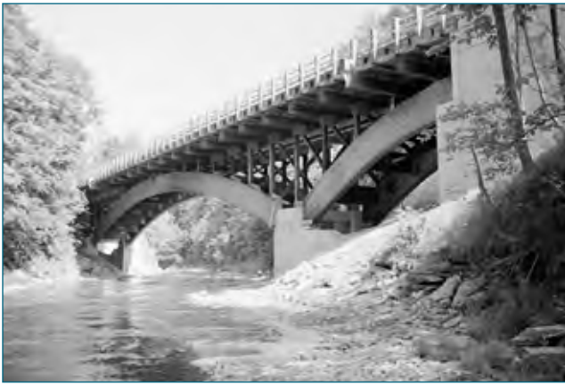
Figure 17–10. The Alton Saylor Memorial Bridge is a glulam deck arch bridge crossing Joncy Gorge in Angelica, New York. The center three-hinged arch spans 52 m (171 ft) and is the longest clear span in the United States. (Photo courtesy of Laminated Concepts, Inc., Big Flats, New York.)
