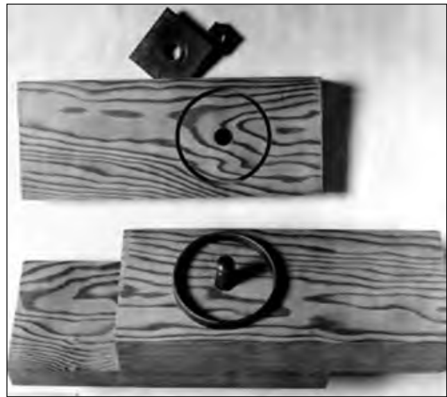
Figure 8–16. Joint with split-ring connector showing connector, precut groove, bolt, washer, and nut.
