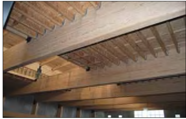
Figure 11–1. Wood-based composites used in the new Centennial Research Facility at the Forest Products Laboratory. Glulam timbers support composite I-joists and plywood sheathing. (Photo by Steve Schmieding, Forest Products Laboratory.)
