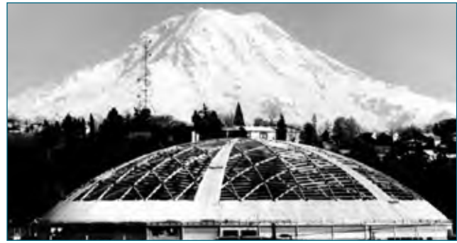
Figure 17-8. This 161.5-m- (530-ft-) diameter Tacoma dome (Tacoma, Washington), built in 1982–1983, is one of the longest clear roof spans in the world. (Photo courtesy of Western Wood Structures, Inc., Tualatin, Oregon.)
