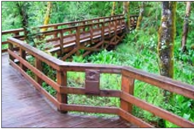
Figure 15–7. Wood preservative leaching, environmental mobility, and effects on aquatic insects were evaluated at this wetland boardwalk in western Oregon.
