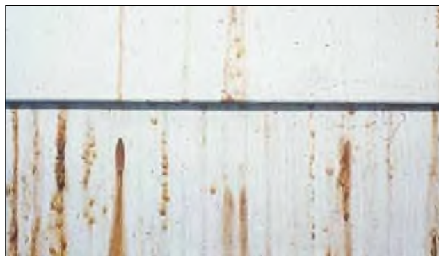
Figure 16–26. Water-soluble extractive discoloration can result from water wetting the back of the siding and then running down the front of the board.
