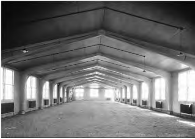
Figure 11–14. Erected in 1934 at the Forest Products Laboratory in Madison, Wisconsin, this building is one of the first constructed with glued-laminated timbers arched, designed, and built using engineering principles.
