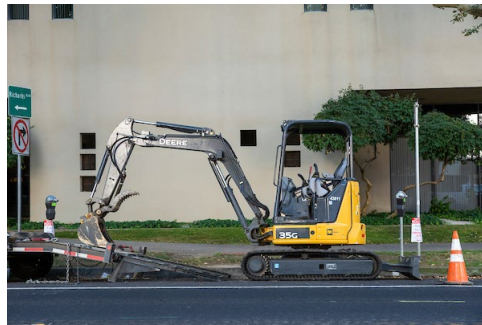
Figure 21. Photo of Excavator
