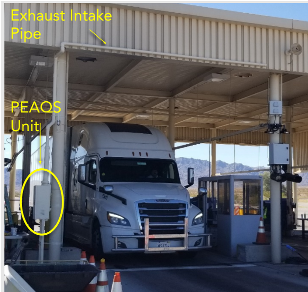
Figure 5-2. Unattended PEAQs system in operation.
