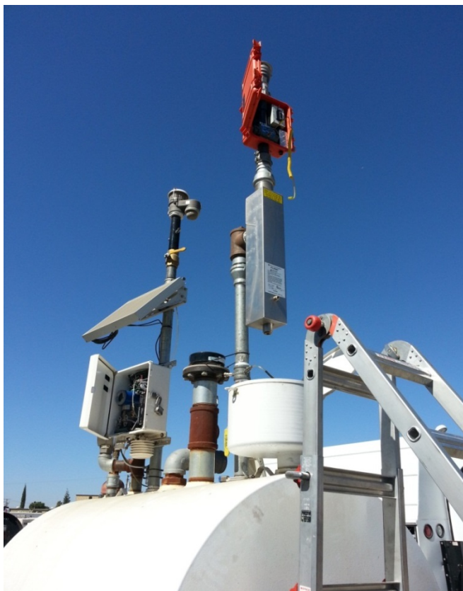
Figure 6: Installation of PV-Zero and Flow Meter
