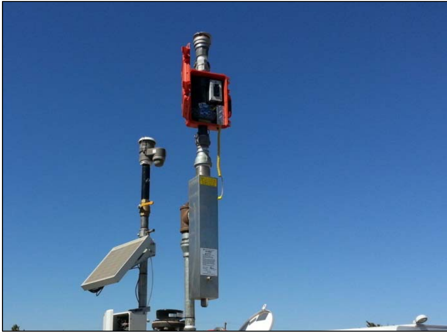
Figure 1B: Typical Installation of PV-Zero on Single Wall AST (with vapor meter above)
