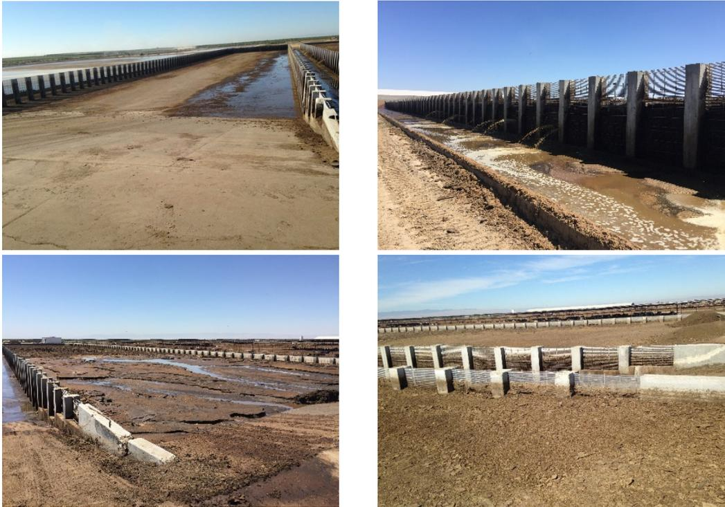
Figure 3-1. Weeping wall cells: empty with an entry ramp (top left), being filled and drained cell (top right), filled cell (bottom left), and filled and dried before emptying (bottom right)
