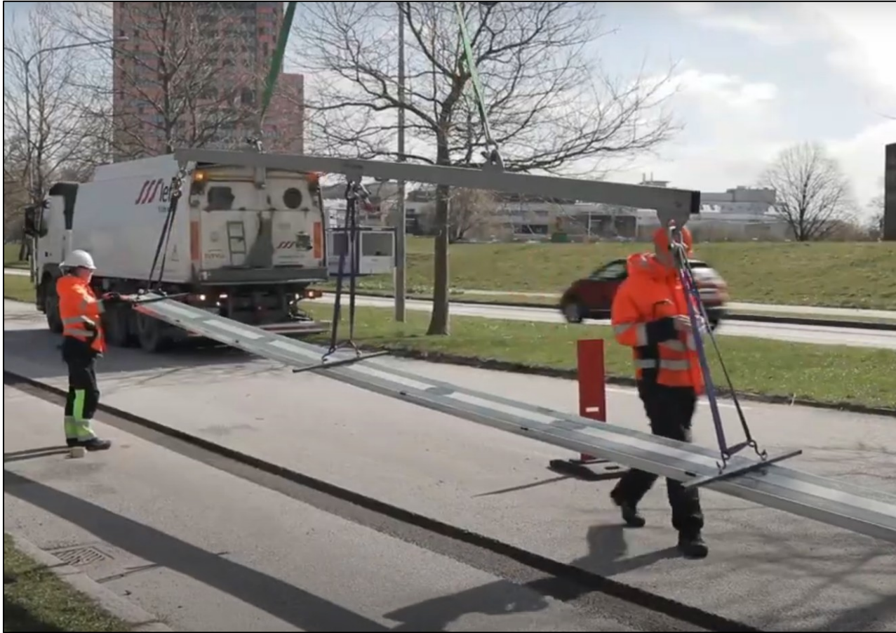
Figure 50: Installation of Charged Track (Elonroad)
