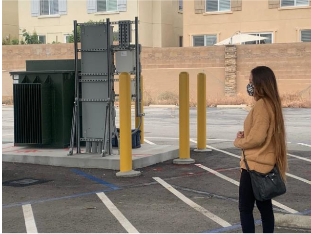
FIGURE 10: CLEAN ENERGY FELLOW WENDY SANCHEZ AT PROJECT SITE
