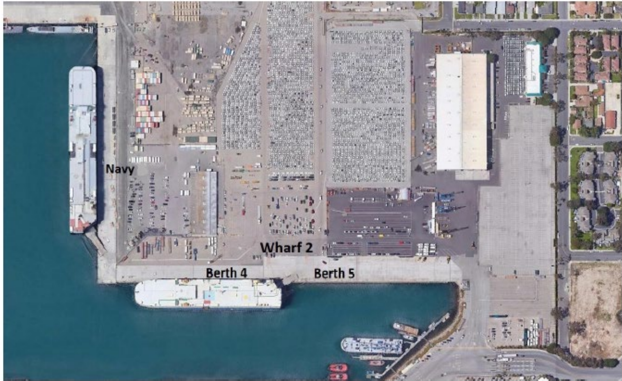
Figure 5.-1: Port of Hueneme North Terminal (Wharf 2)
