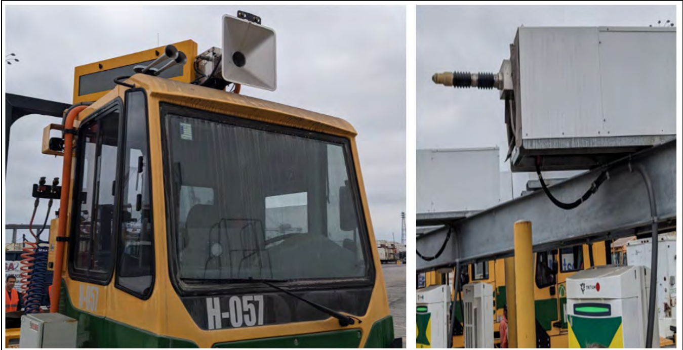
Figure 45: Hands-Free Conductive Charging System (Staff photo)
