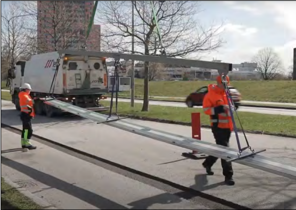
Figure 49: Installation of Elonroad Charged Track (Elonroad)
