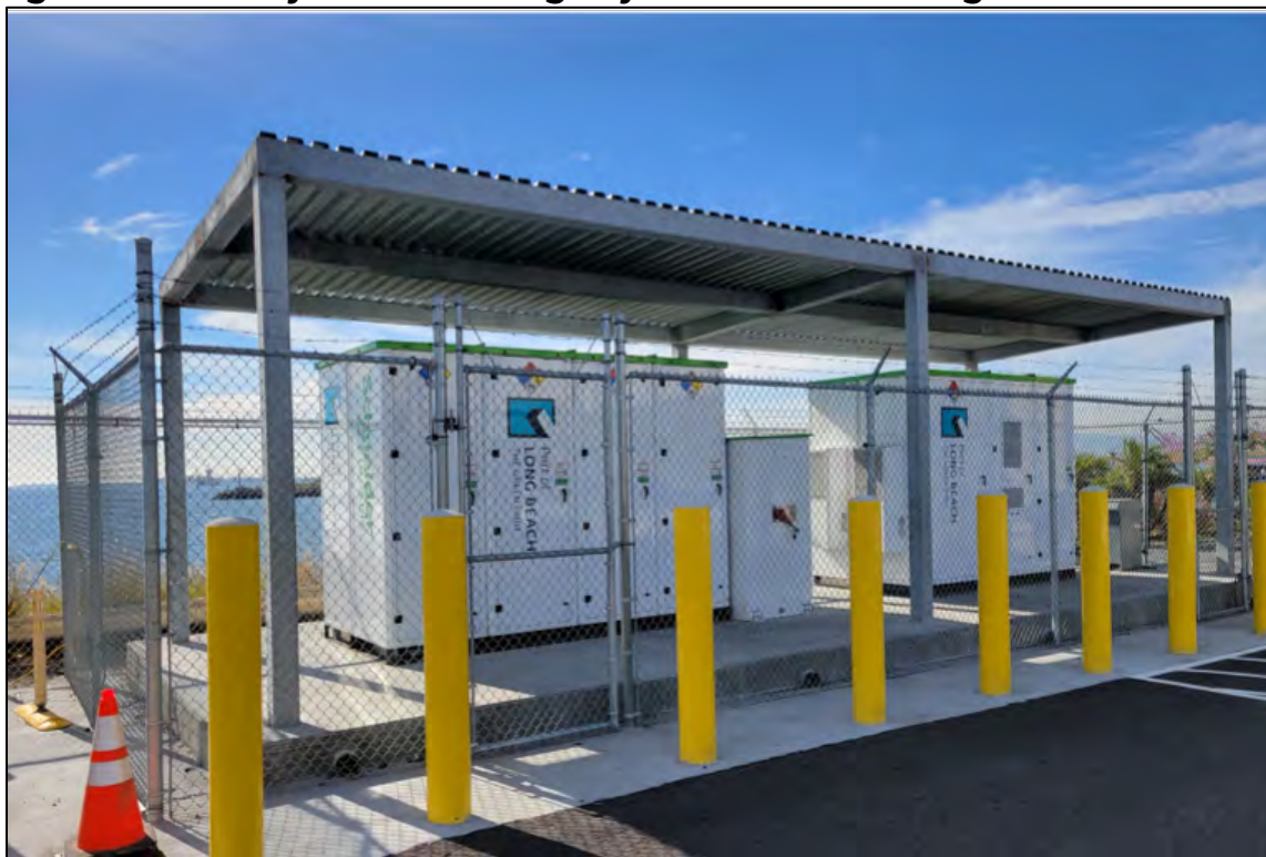
Figure 42: Battery-Electric Storage System at Port of Long Beach 100
