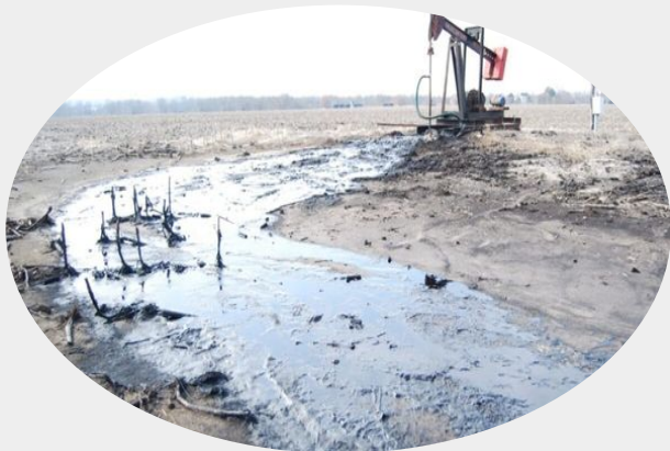
Fixing Abandoned Wells
