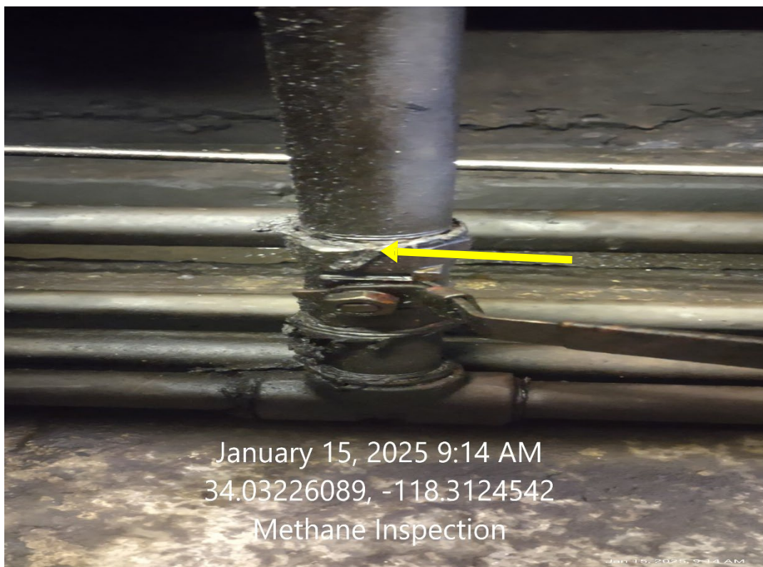
Figure 3: Photograph of the identified leak location on Well Murphy #5
