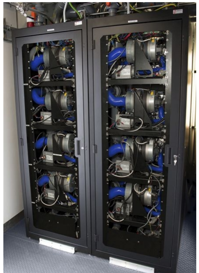
Hydrogen Fuel Cell Rack Assembly
