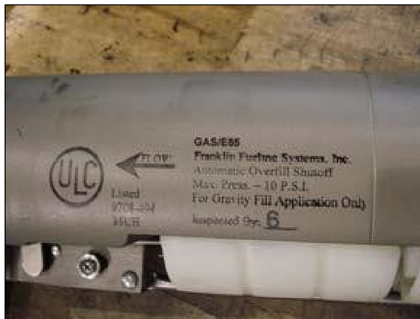
EBW 70849X3Y Autolimiter (Gas/E85 Compatible)
