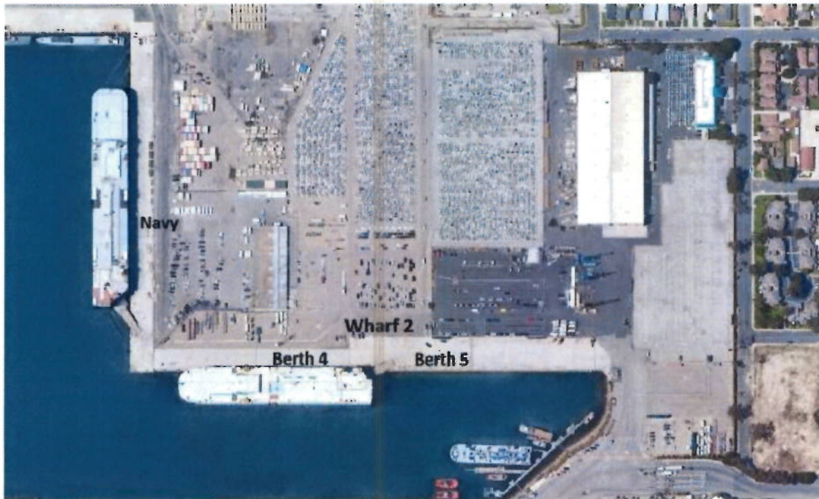
Figure 5-1: Port of Hueneme North Terminal (Wharf 2)
