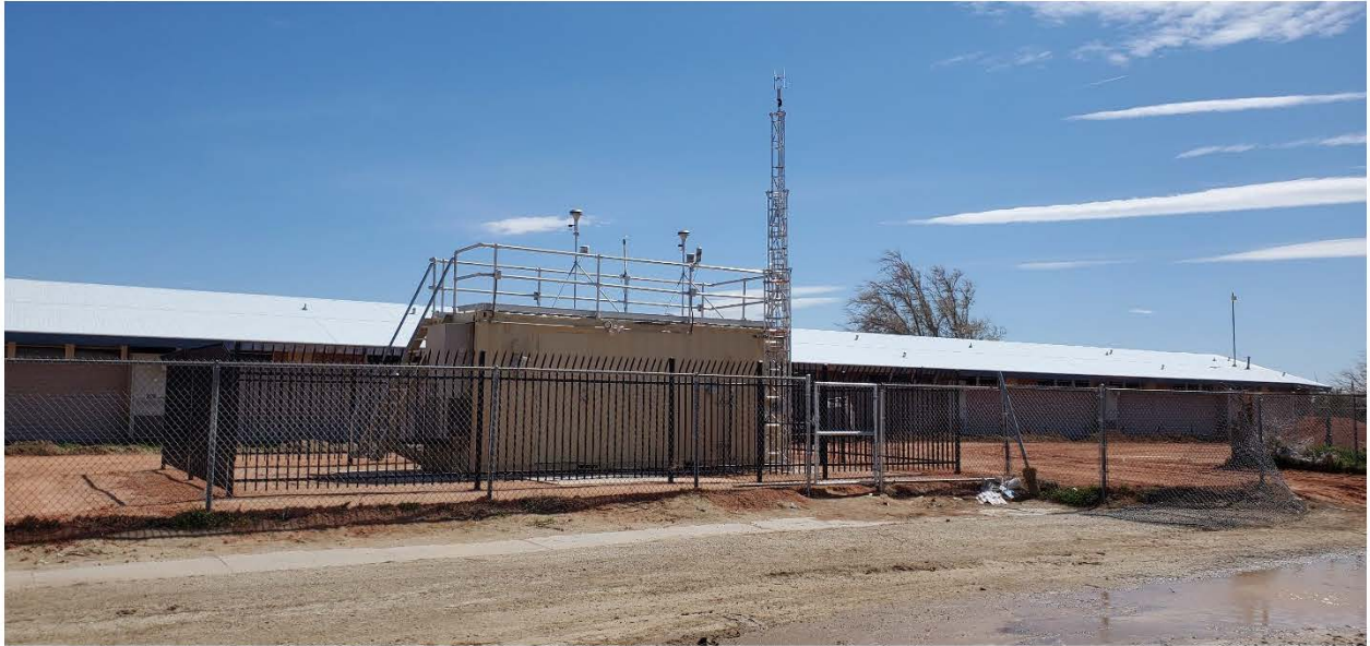
Photo 1: Pat Avenue Shelter
