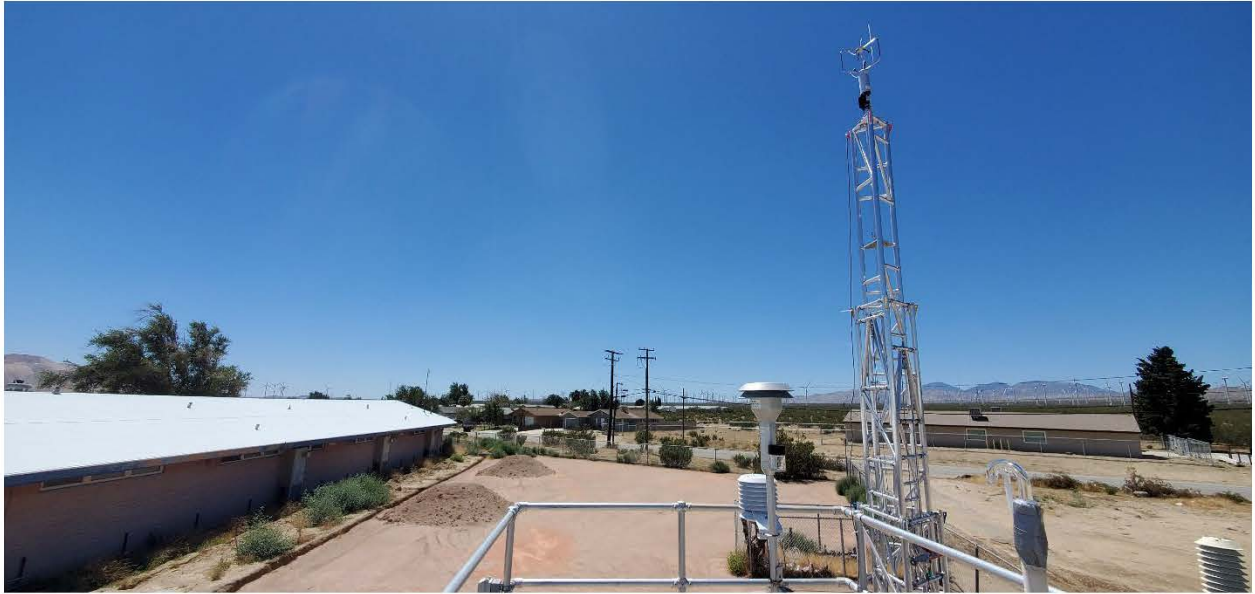
Photo 2: Pat Avenue Shelter, Rooftop West View
