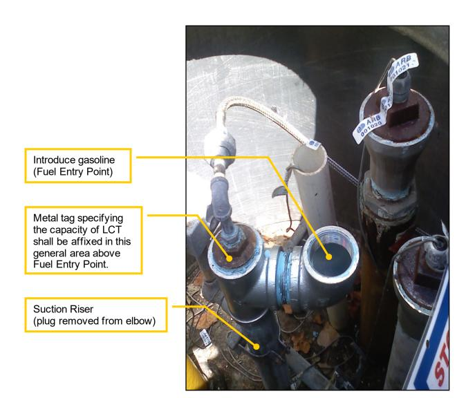
Figure 3 Adding Gasoline through Open Fuel Point
