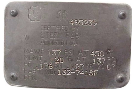
Clean Air Separator Data Plate (not pictured on far side of base)
