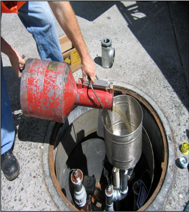
FIGURE 16-3 Adding Gasoline through Open Fuel Point
