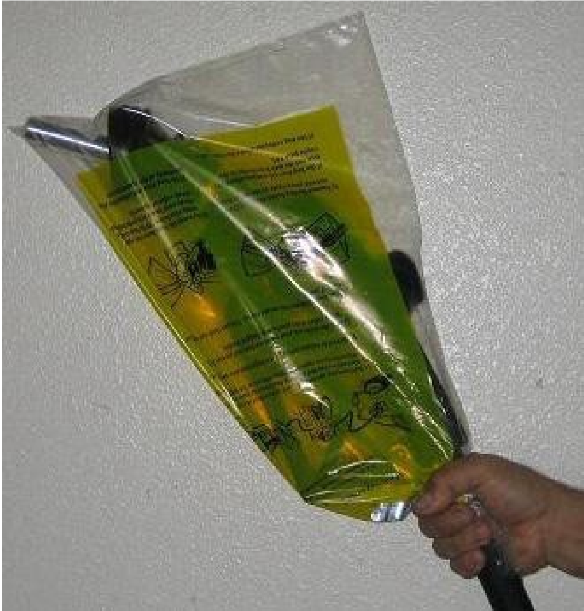
FIGURE 7-1 Typical Example of Bagging a Nozzle
