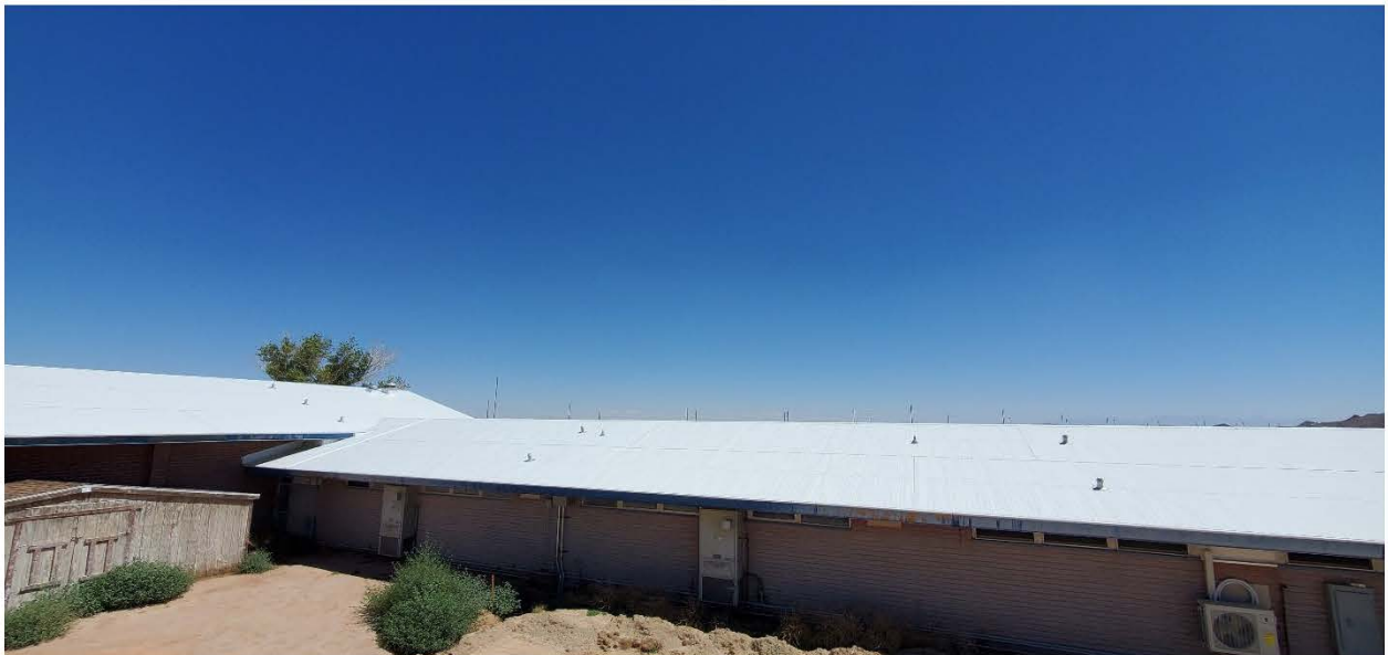
Photo 4: Pat Avenue Shelter, Rooftop South View
