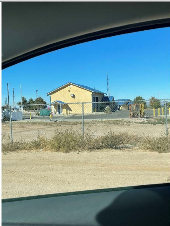
Figure 16 - Cal Fire Above Ground Storage Tank
