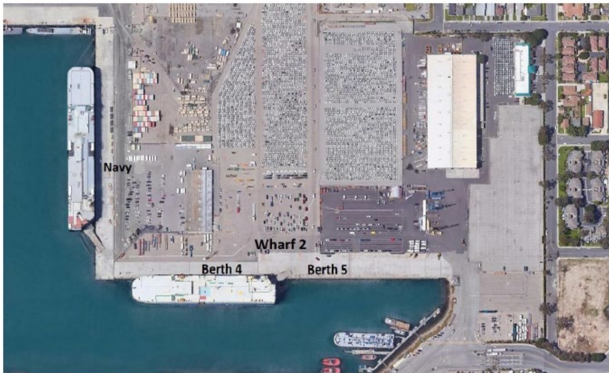
Figure 5-1: Port of Hueneme North Terminal (Wharf 2)
